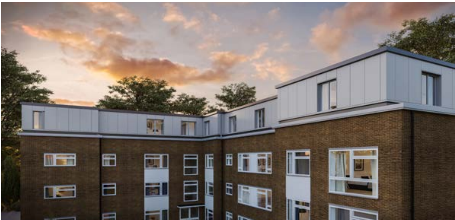
Above: The View, Putney SW11- an airspace development above an existing residential block.
